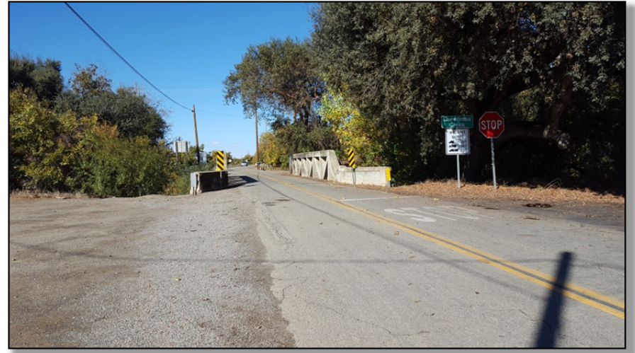
View northwest at Kilburn Road Bridge.
