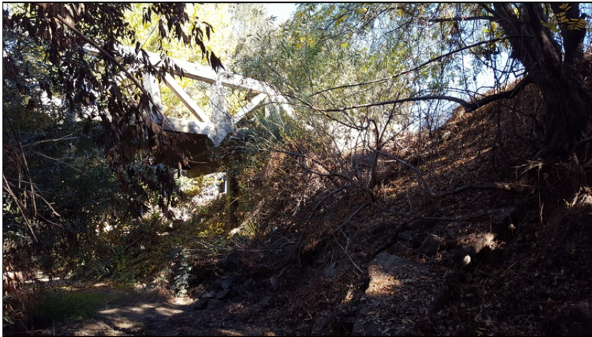
View of eastern end of Kilburn Road Bridge from Orestimba Creek bed.
