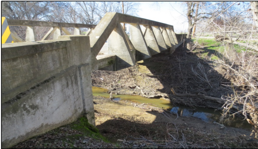
View west at Kilburn Road Bridge over Orestimba Creek.
