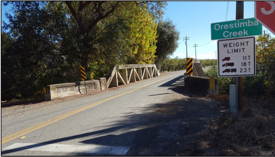
View east at Kilburn Road Bridge.
