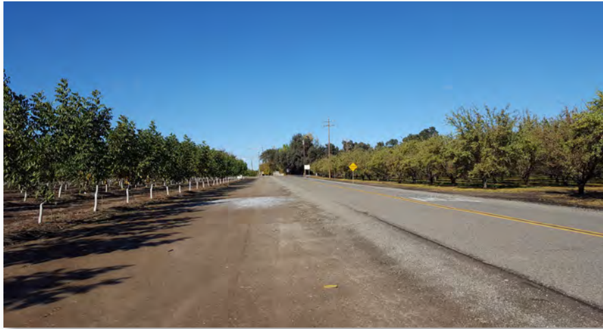
East side of Kilburn Road bridge looking west towards bridge.
