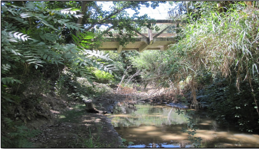
View southwest at Kilburn Road Bridge from Orestimba Creek bed.
