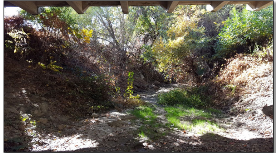
View northeast at Orestimba Creek bed from underneath Kilburn Road Bridge.
