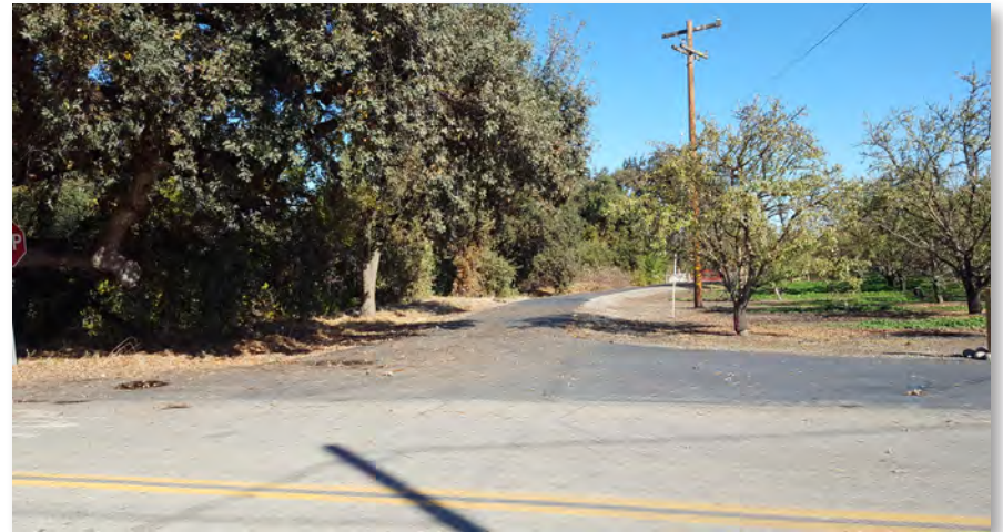
East side of the Kilburn Road bridge looking north.
