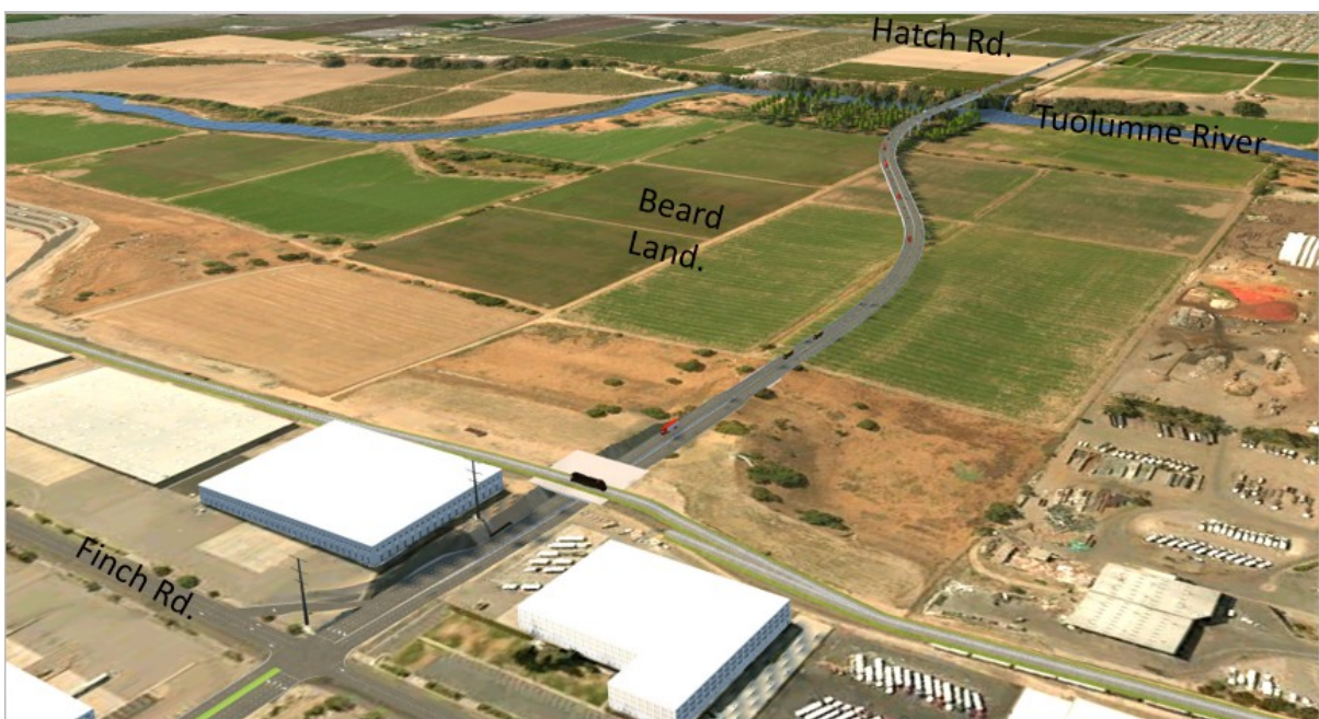
Figure 2.2-9. Aerial view looking south after improvements.
