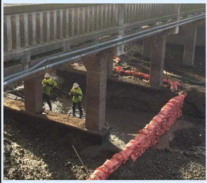
is the removal of sediment such as sand and rocks from around bridge abutments or piers. Scour, caused by swiftly moving water, can scoop out scour holes. compromising the integrity of a structure.
