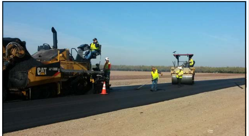
Asphalt Overlay
