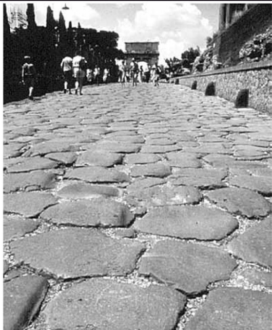
Figure 1. The Roman Appian Way: early interlocking pavement
