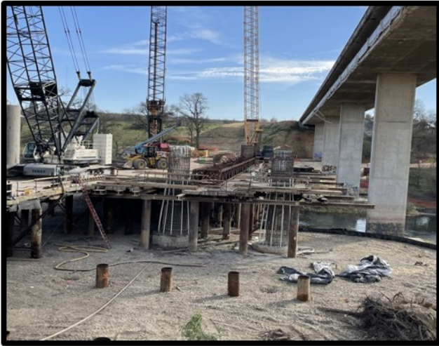
Construction of the new bridge base
