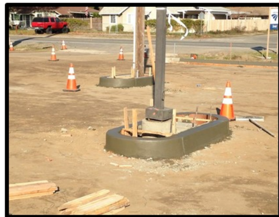
Fresh cement curb for new additional lighting.
