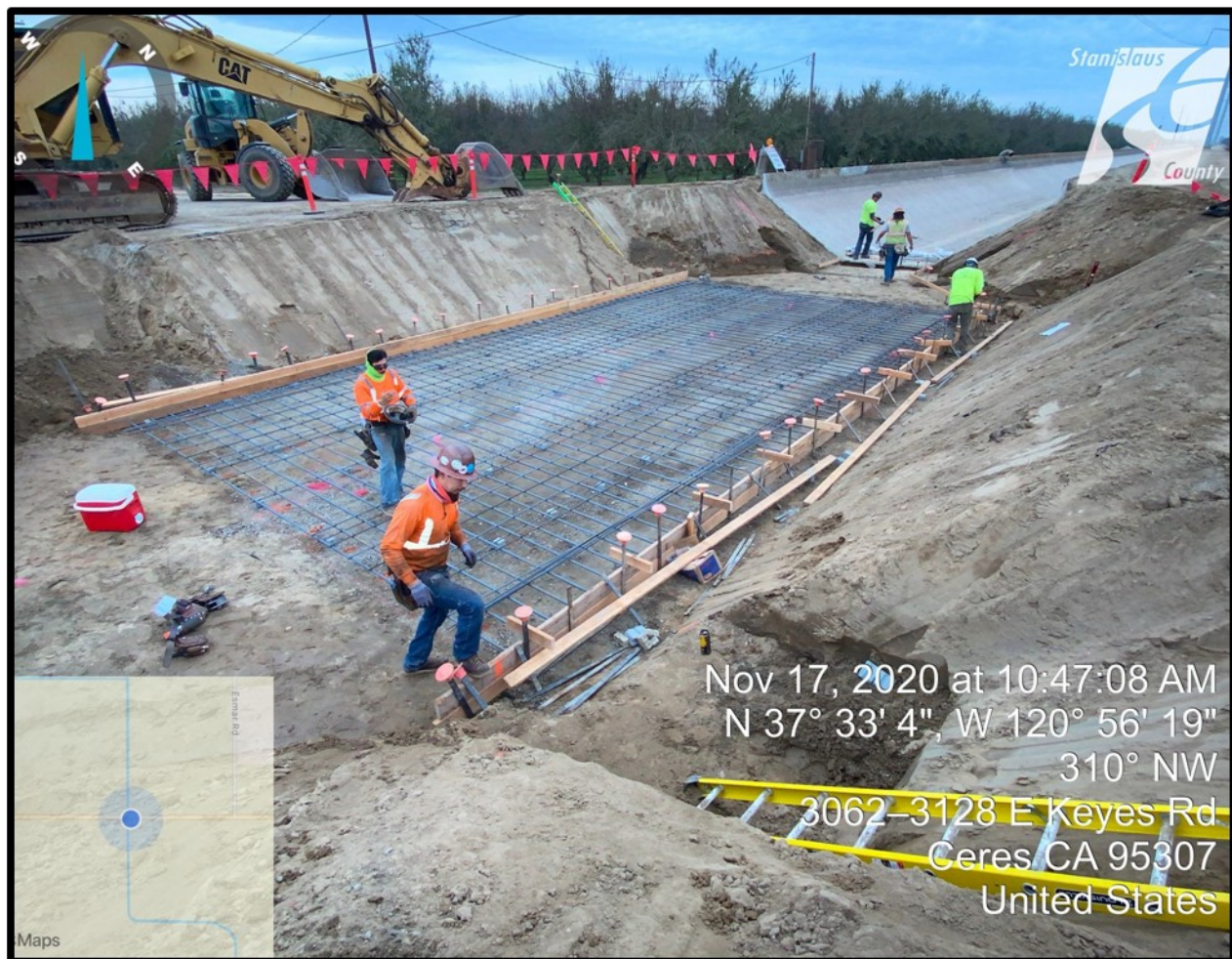
Stanislaus County workers laying the new canal foundation for the future new bridge.
