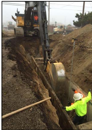
Checking Grade on Kerr Avenue
