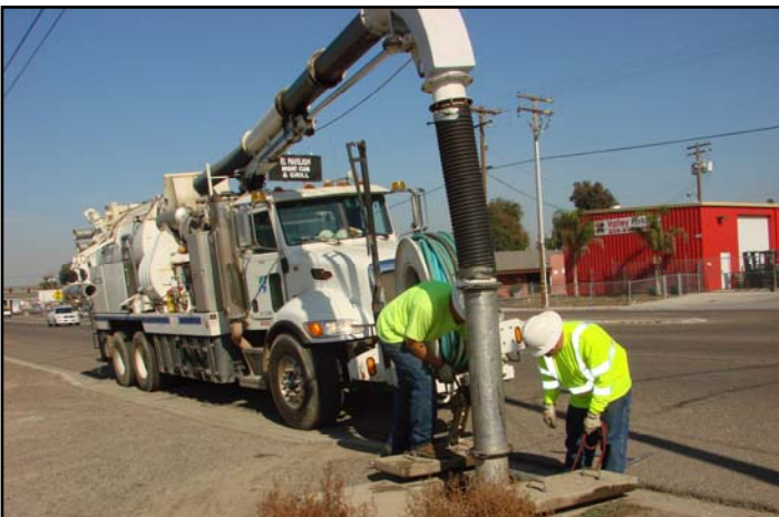
Road Maintenance Workers James Sanchez and Steuart Holt operating the vacuum cleaning drains on 9 th Street in Modesto
