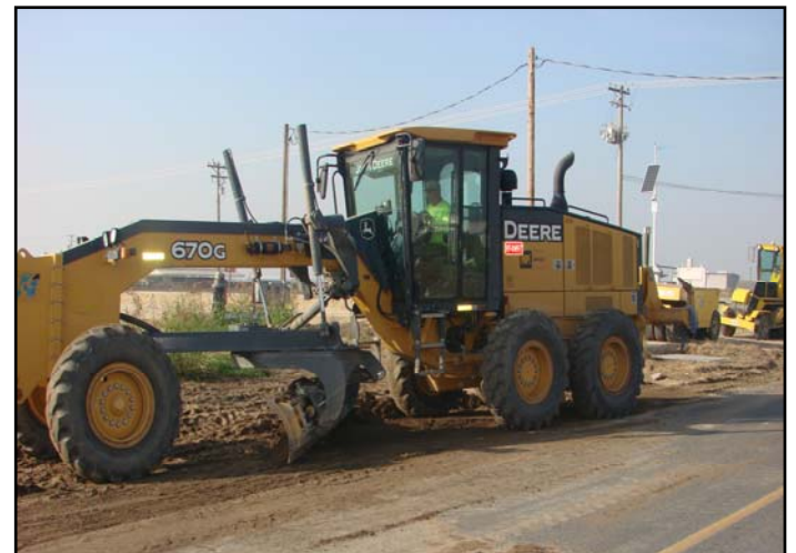
George Molina, Road Maintenance Worker is operating grader to smooth out a new shoulder on Ehrlich in Turlock
