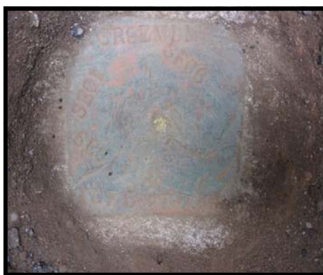
This is a section corner on Faith Home Road. It is a 10" diameter concrete monument that was set in 1904. It now has a 2" iron pipe on top with a monument well at road level, and will possibly never be seen again.
