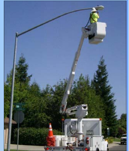
Replacing an old high pressure sodium street light to the new induction lighting head.
