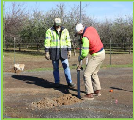
Larry and Scotty set a monument to re-establish the section corner.
