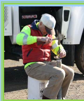
Scotty stamping monument cap with section township, range information, and County Surveyor Wayne Sutton's Land Surveyor number.
