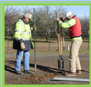
Digging section corner position notice 4' x 2" I.P. laying on ground
