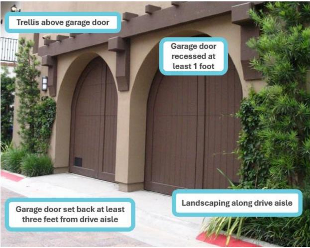
Figure 9 Garage Door Design Features
