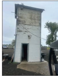
EXISTING WELL HOUSE - EAST
