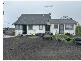
EXISTING HOUSE - SOUTH
