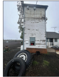
EXISTING WELL HOUSE - SOUTH
