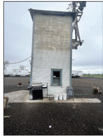
EXISTING WELL HOUSE - NORTH
