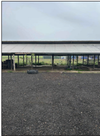
EXISTING CORRAL - NORTH
