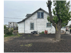
EXISTING HOUSE - WEST
