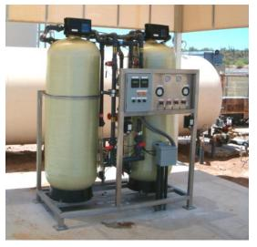
Use of E33 media in typical Adsorption Package Units (APU) and Modular System installations).
