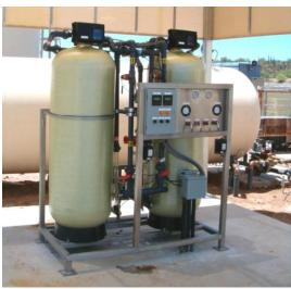
Use of E33 media in typical Adsorption Package Units (APU) and Modular System installations).
