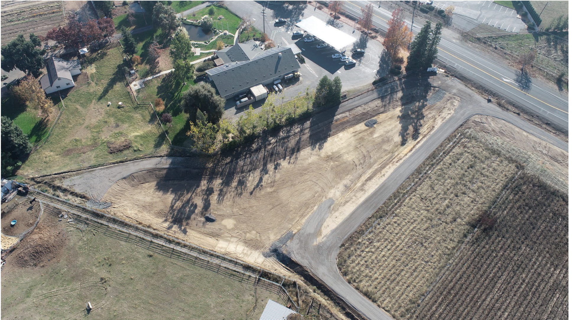
AERIAL VIEW OF DRAINAGE BASIN SHOWING SR 120 FRONTAGE
