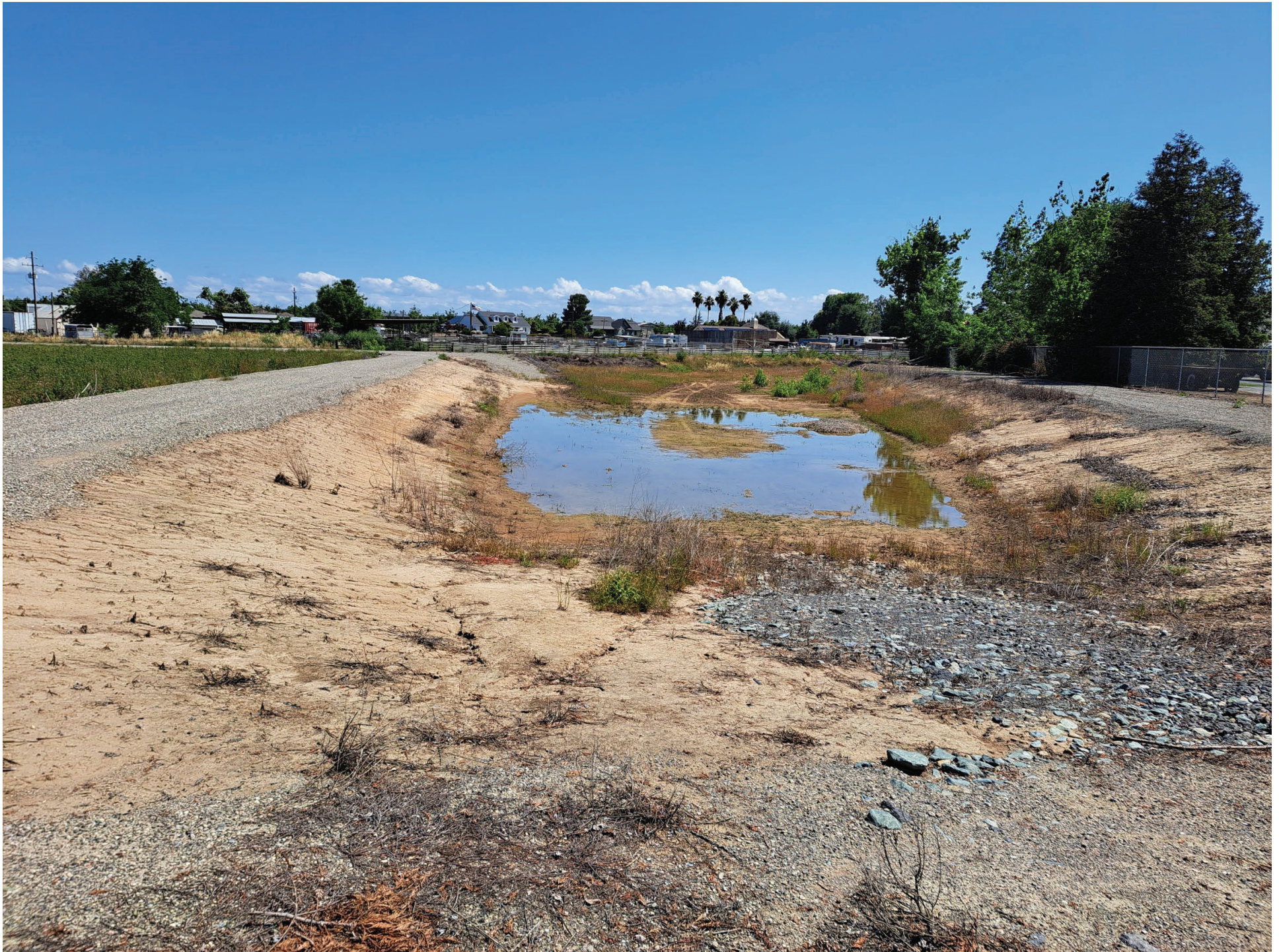
VIEW LOOKING NORTHEAST TOWARD PROPOSED PARCEL 1, SHOWING DRAINAGE BASIN
