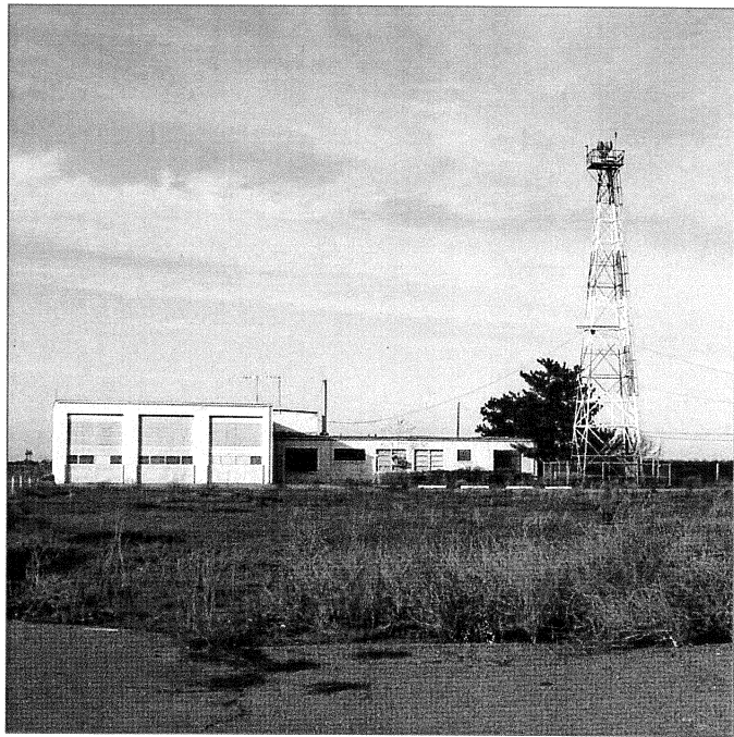
Abandoned military facilities at former Crows Landing Air Facility.
