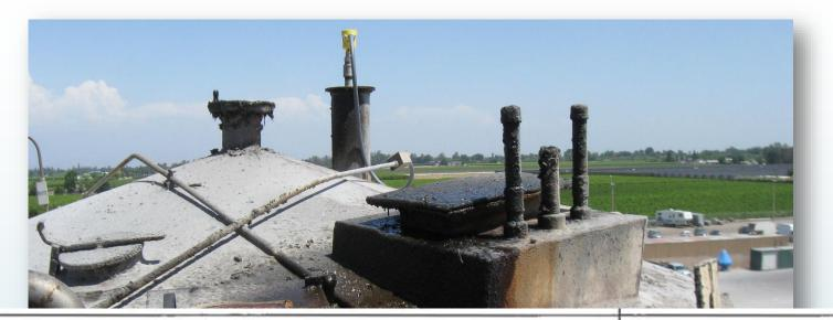
Is overfill prevention equipment in good working condition? If it is equipped with a mechanical test mechanism, actuate the mechanism to confirm operation.
