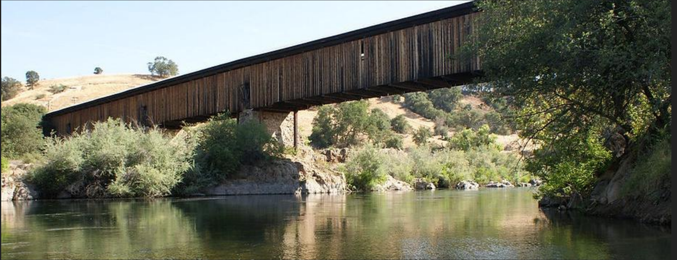
Photo Credit: Knights Ferry Bridge, https://knightsferry.com/
