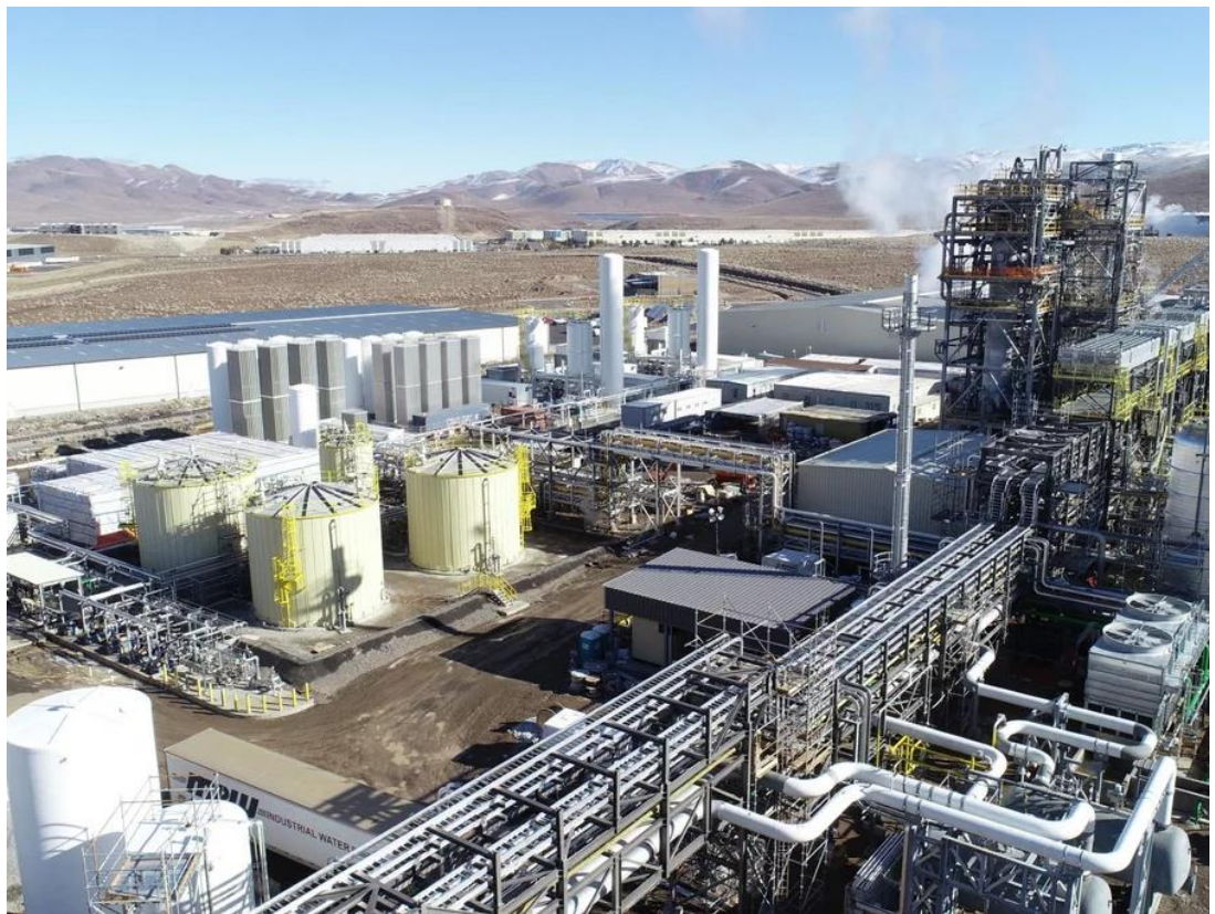
Figure 8. Fulcrum Sierra Biofuels Facility
