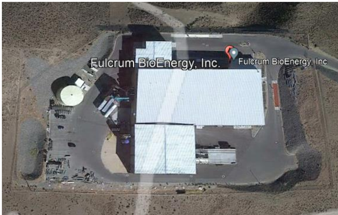
Figure 6. Fulcrum BioEnergy Feedstock Preparation Facility (FPF)
