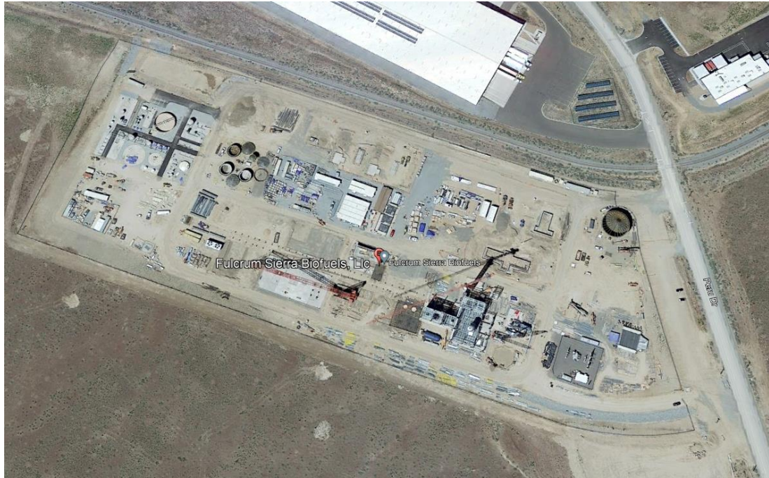
Figure 7. Fulcrum Sierra Biofuels Facility (Aerial)
