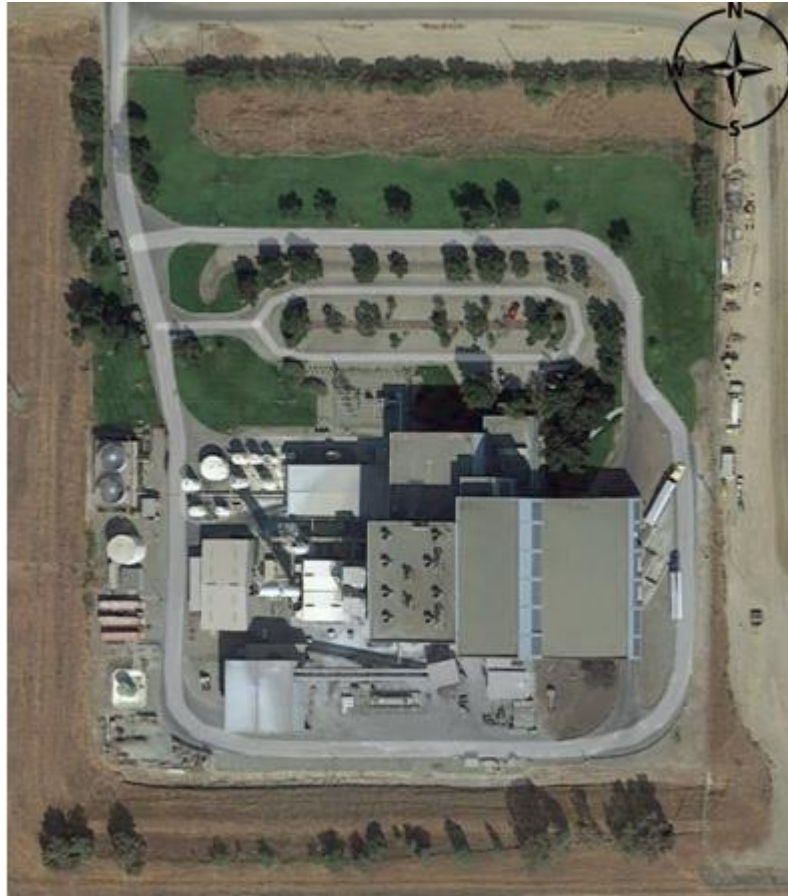
Figure 3. Covanta WTE Facility in Stanislaus County (Aerial)
