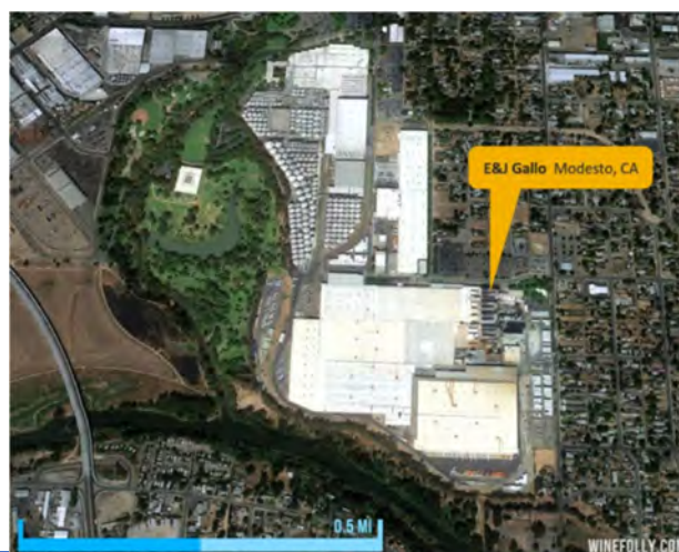
E. & J. Gallo Winery headquarters, Modesto
