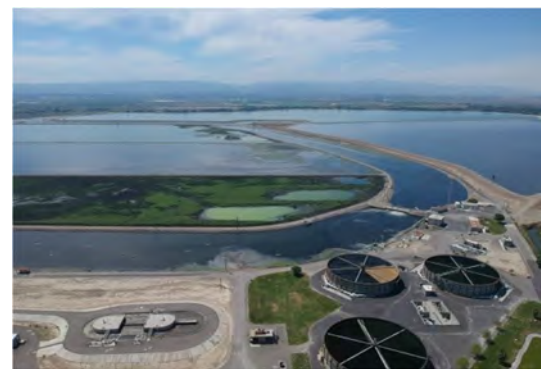
Modesto's Jennings Water Treatment Plant
