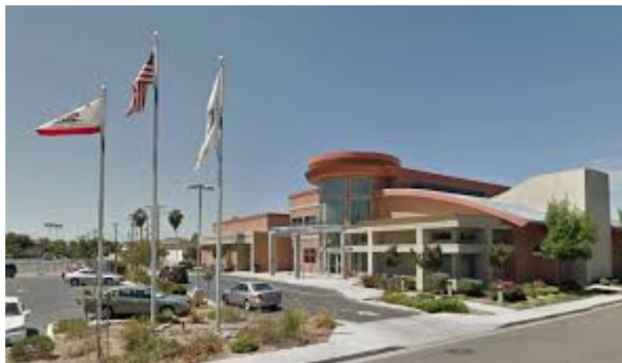
Photo 12- Ceres Community Center
