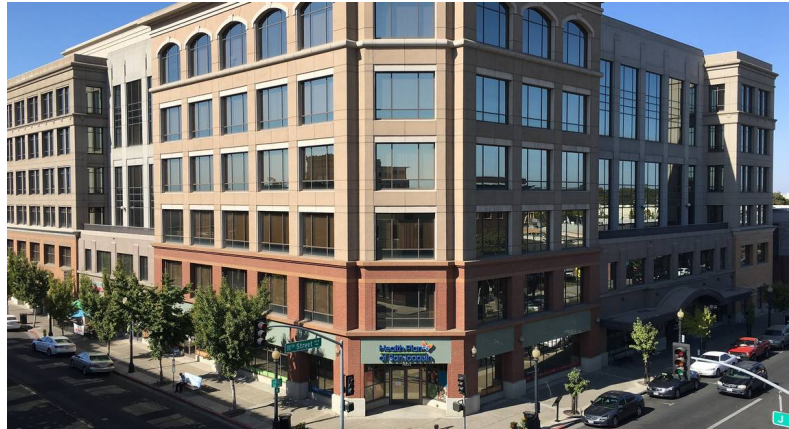
Photo 1- Tenth Street Place
