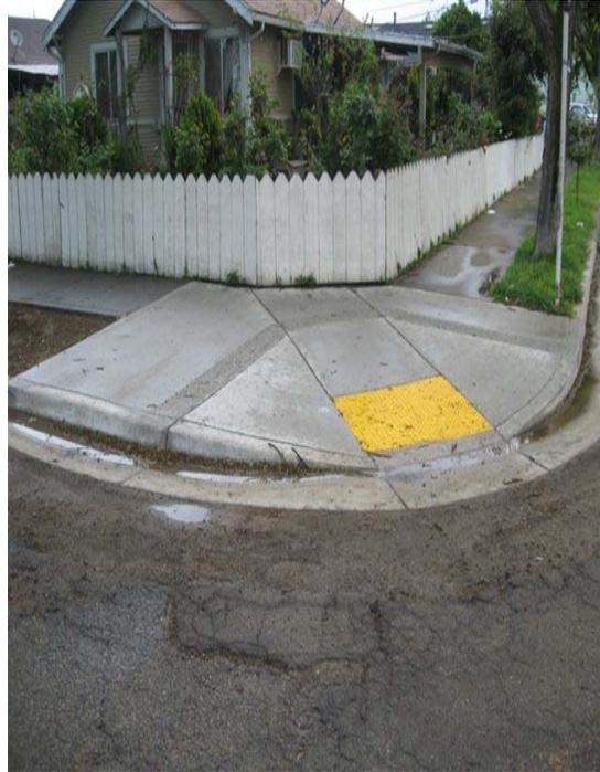
Photos reflect 3<sup>rd</sup> Street ADA accessible ramp installations.
