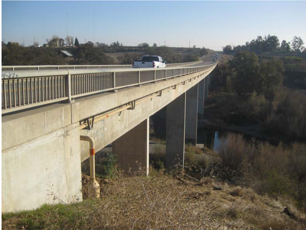
PHOTOGRAPH 3: Gas pipeline on west side of bridge.
