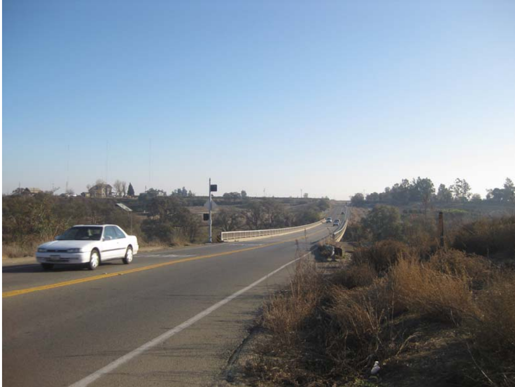
PHOTOGRAPH 1: Hickman Road and Bridge, facing south.
