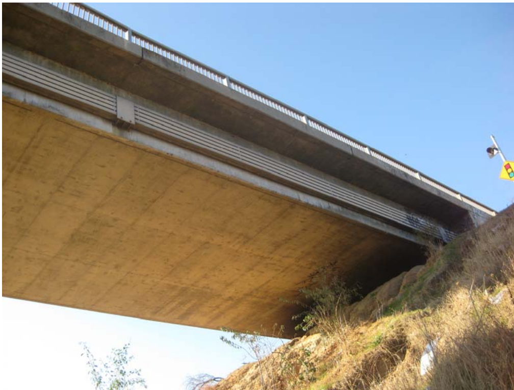
PHOTOGRAPH 4: Electrical utilities on east side of bridge.
