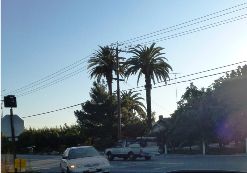
View from Claribel Road at Coffee Road intersection looking southwest at 4929 Coffee Road. Photo 19 October 2012.
