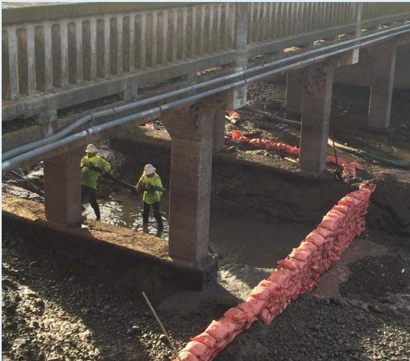
*Bridge scour is the removal of sediment such as sand and rocks from around bridge abutments or piers. Scour, caused by swiftly moving water, can scoop out scour holes, compromising the integrity of a structure.*
