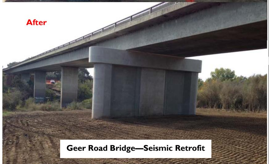
Geer Road Bridge—Seismic Retrofit
