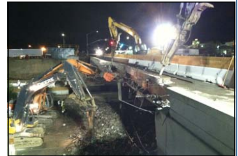
Box culvert construction slab poured in late December 2013
