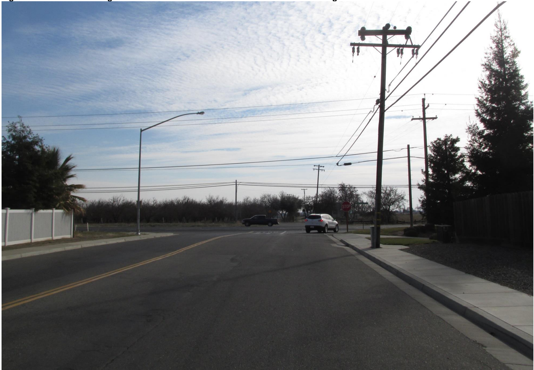
Figure 3.1.7-6: KV-7 Existing Condition - From Atlas Road and SR-108/SR-120 Looking South
