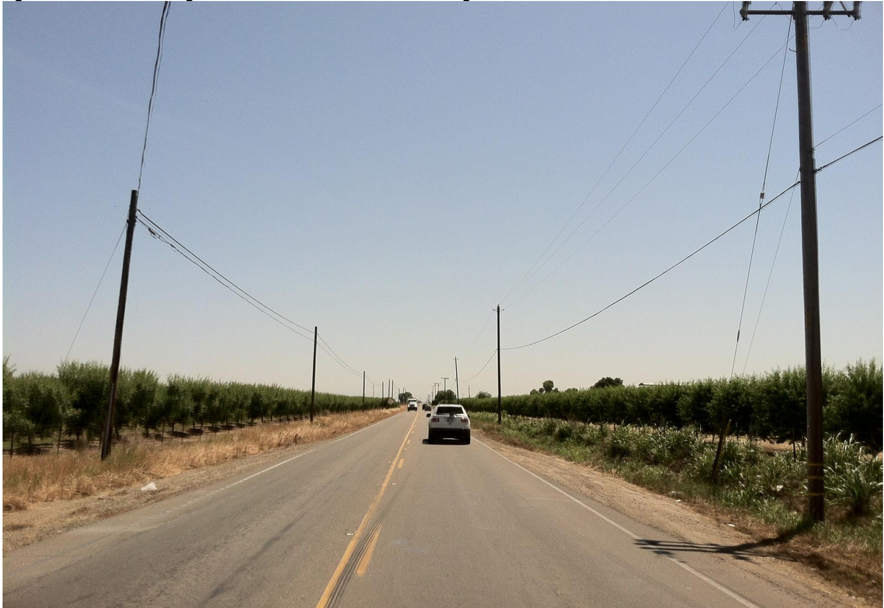
Figure 3.1.7-12: KV-3 Existing Condition – From Patterson Road Looking East
