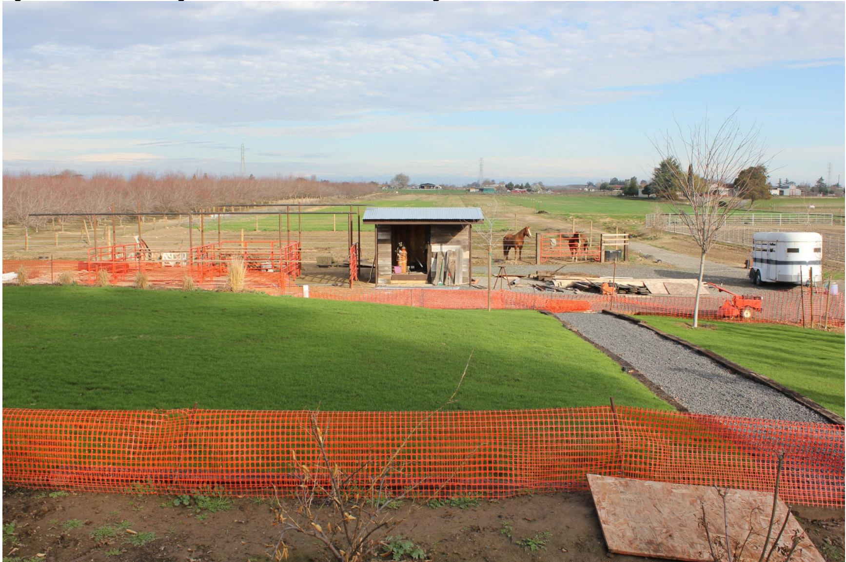
Figure 3.1.7-14: KV-5 Existing Condition - From Townhill Road Looking East
