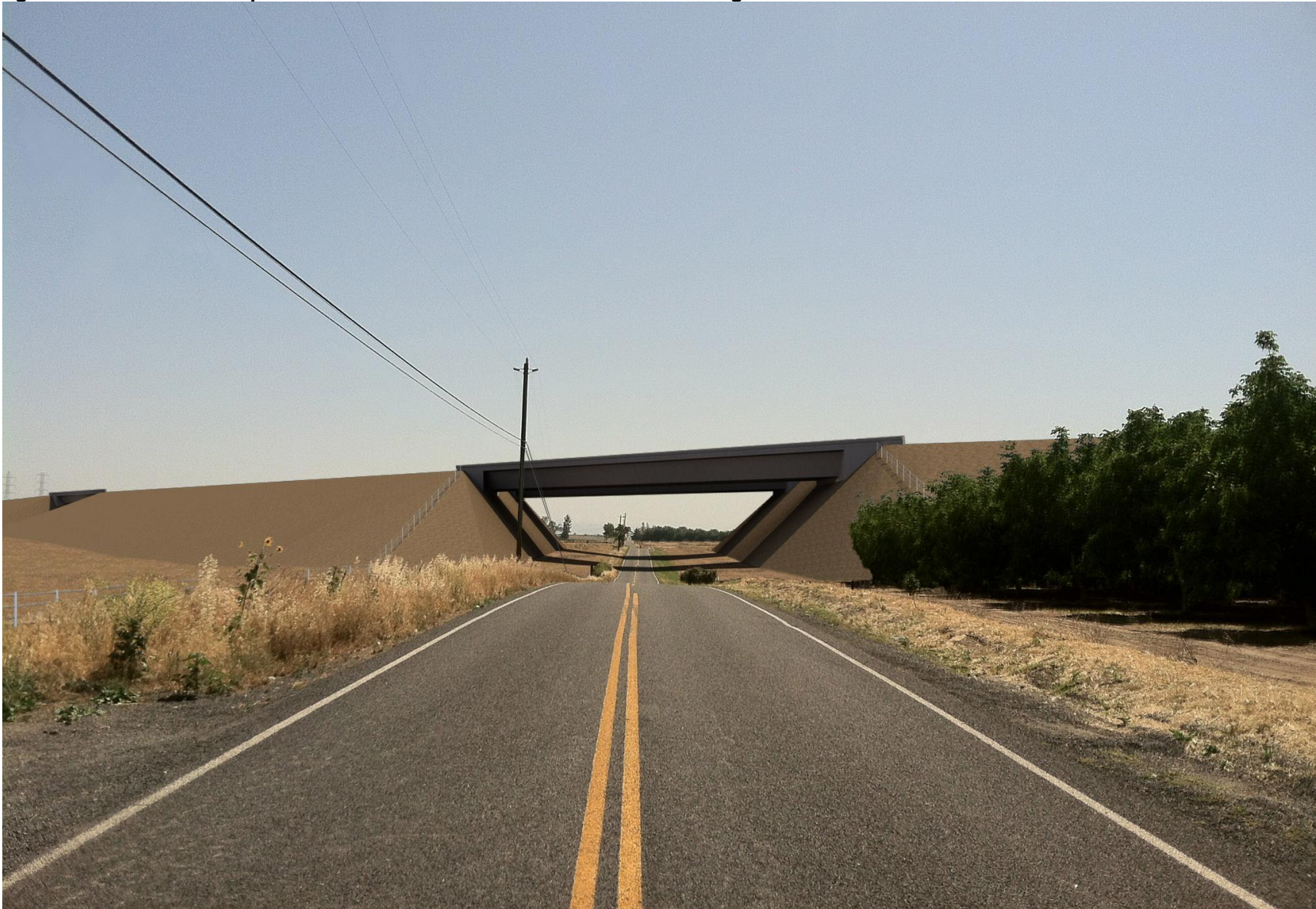
Figure 3.1.7-21: KV-10 Proposed Condition – From Warnerville Road Looking East – Alternative 2B
