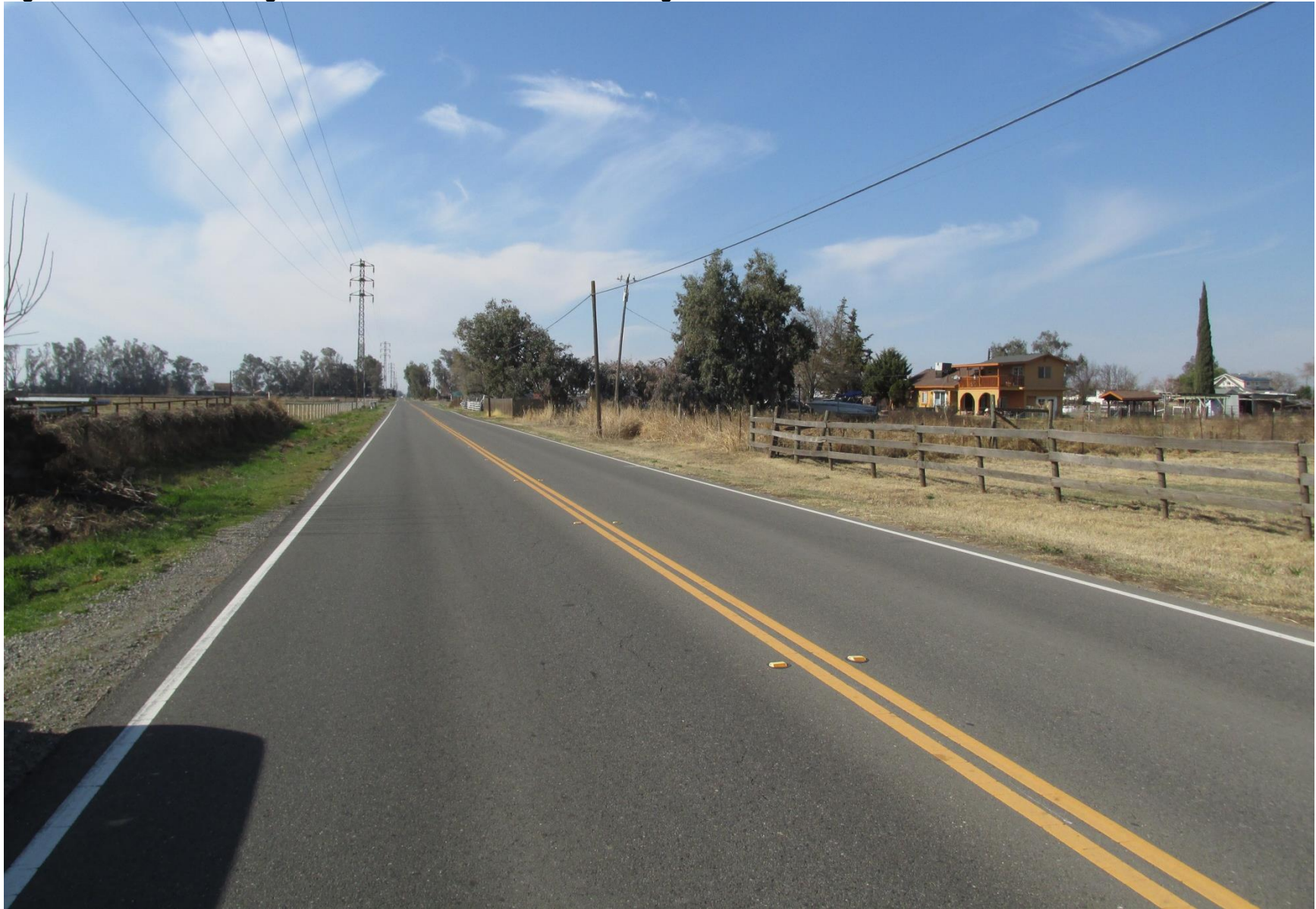
Figure 3.1.7-8: KV-8 Existing Condition -- From Claribel Road Looking West
