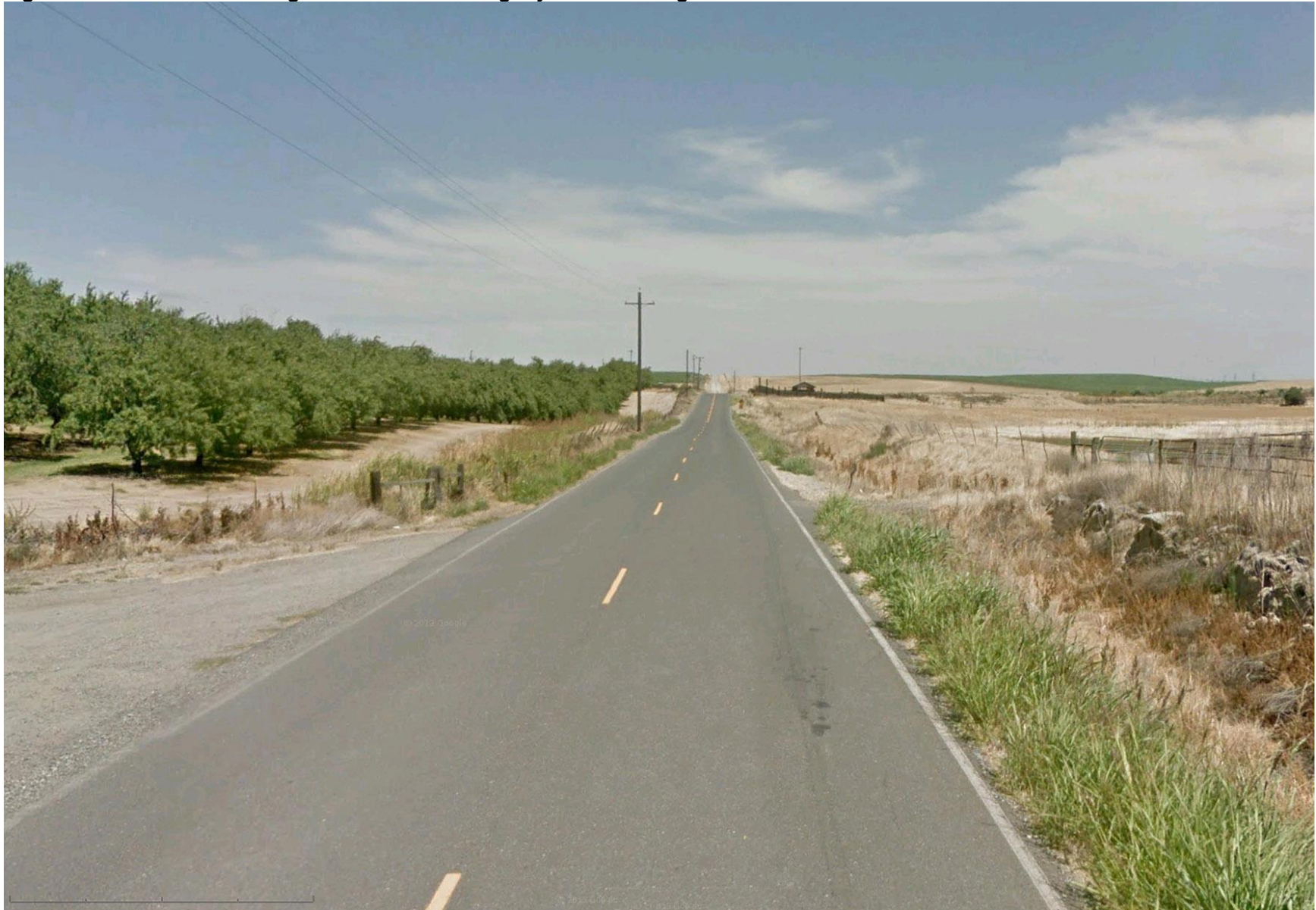
Figure 3.1.7-22: KV-11 Existing Condition - From Fogarty Road Looking East
