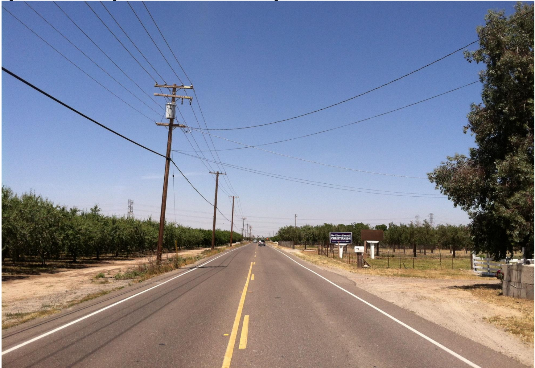
Figure 3.1.7-10: KV-1 Existing Condition – From Oakdale Road Looking North
