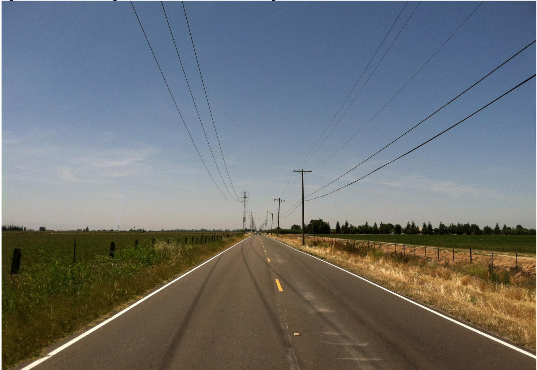
Figure 3.1.7-18: KV-9 Existing Condition - From Claribel Road Looking West
