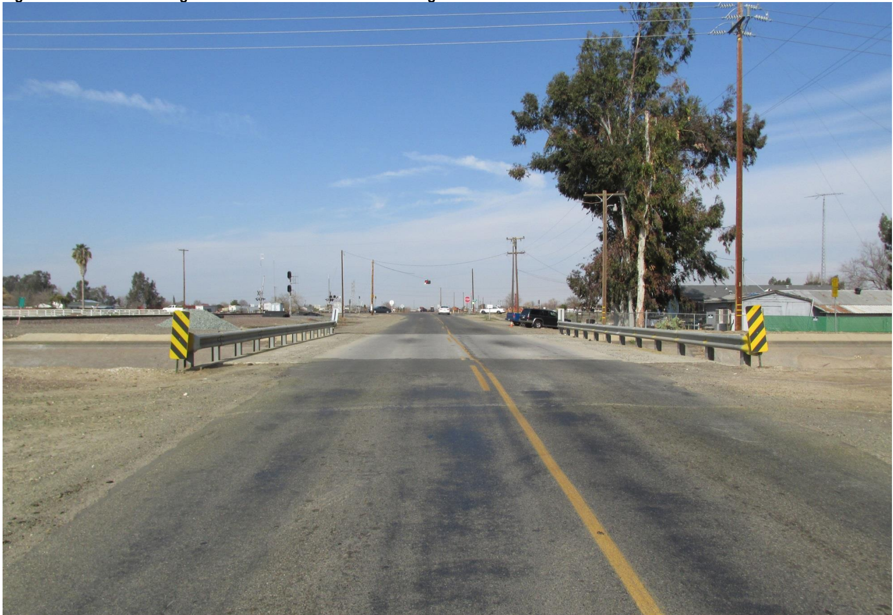
Figure 3.1.7-2: KV-2 Existing Condition - Terminal Avenue Looking North
