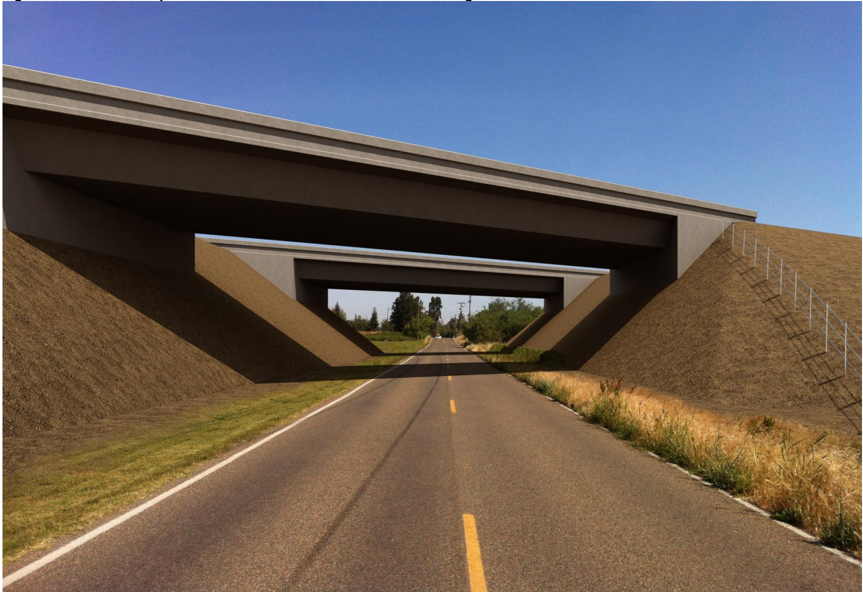
Figure 3.1.7-17: KV-6 Proposed Condition – From S. Stearns Road Looking North – Alternatives 1A and 2A
