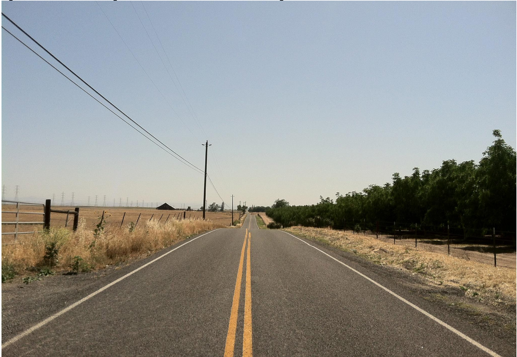
Figure 3.1.7-20: KV-10 Existing Condition - From Warnerville Road Looking East
