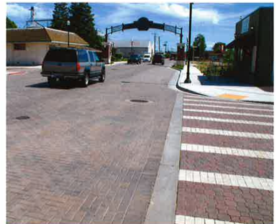
Main Street in historic downtown Ripon features 50,000 sf (4,645 m 2 ) of interlocking concrete pavement.
