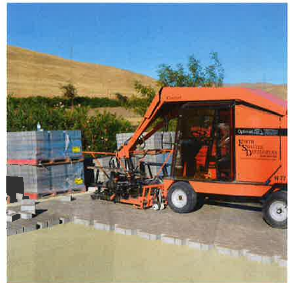
Machine-assisted installation of interlocking concrete pavement in Westley, CA.
