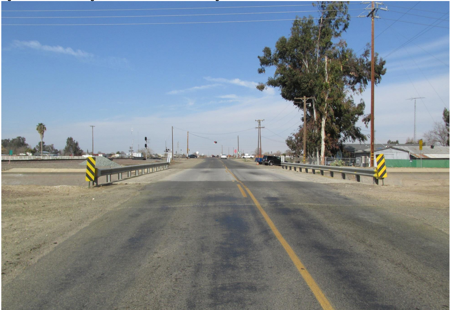
Figure 3.1.7-2: KV-2 Existing Condition - Terminal Avenue Looking North
