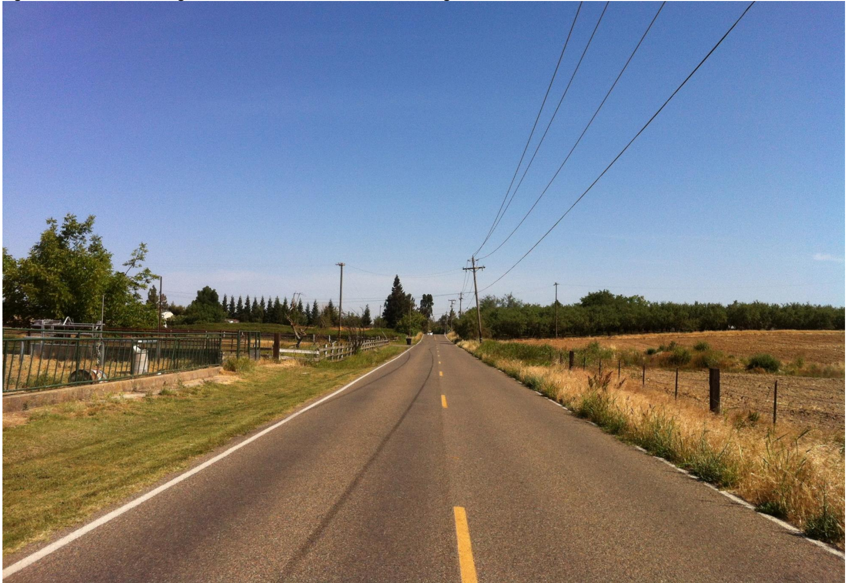
Figure 3.1.7-16: KV-6 Existing Condition - From S. Stearns Road Looking North
