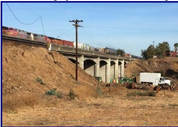
Trees designated for normal removal were removed from an elevation that is six inches above the adjacent ground surface. The stumps and roots were left intact to avoid any ground disturbance. Trees designated as potential bat habitat were removed using the following two-step process, conducted over two consecutive days:
