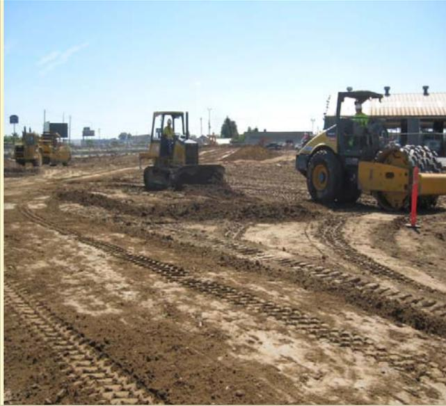
Pictured above are the building pads being graded. Some rough weather slowed this process down quite a bit since soils were saturated.
