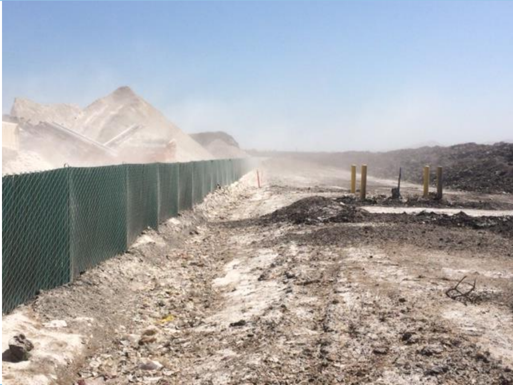
Photograph 7: View from ST-4; facing south
