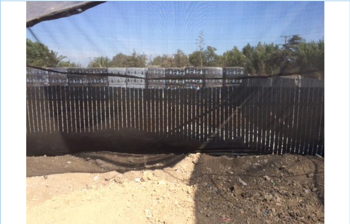
Photograph 2: View from ST-1; facing east
