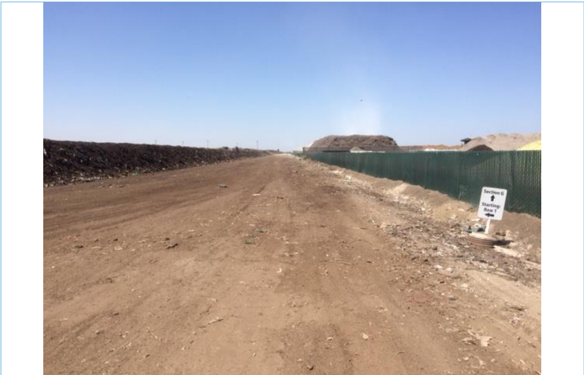
Photograph 1: View from ST-3; facing north
