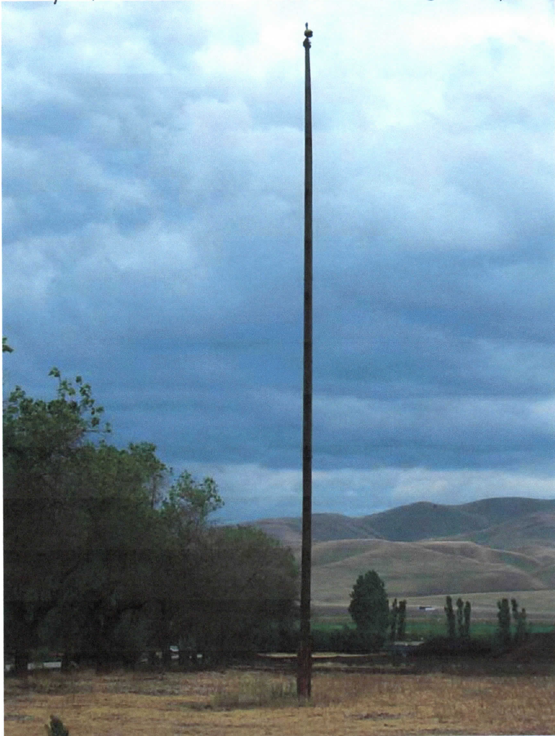
The station's flagpole
