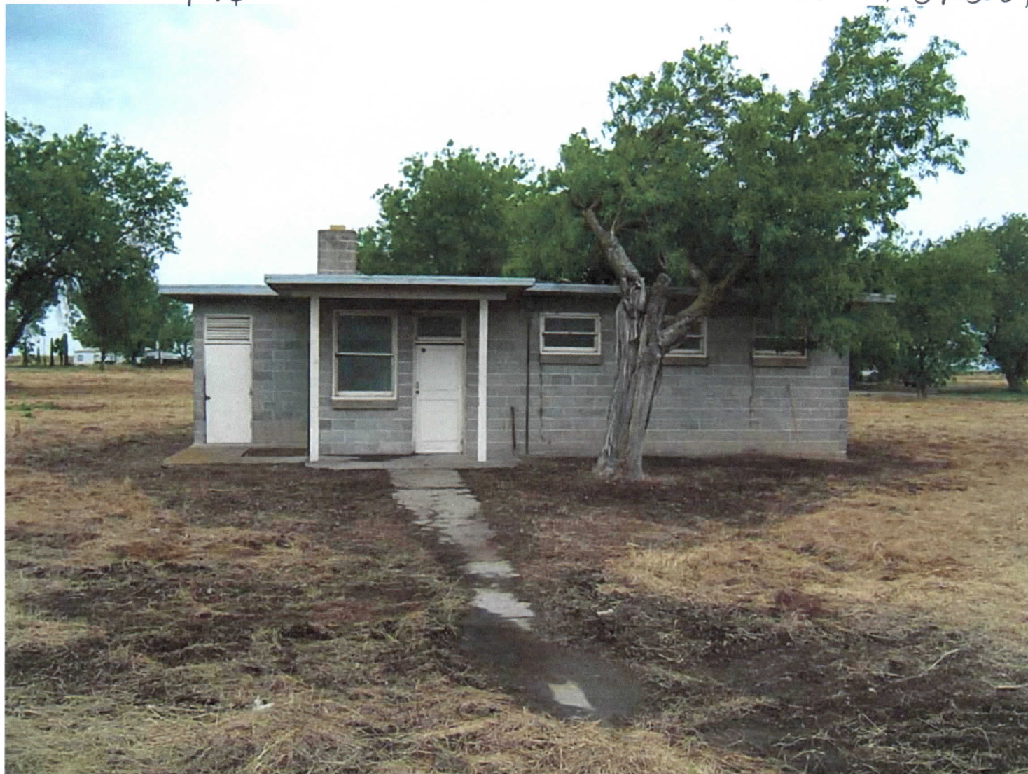
This building is shown on the 1946 station map as the station's brig and according to the owners, the building still has cells inside.
