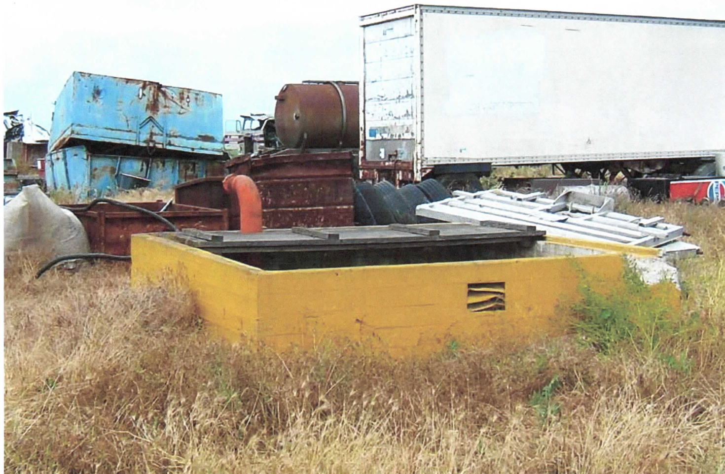
One of three 50,000 gallon underground concrete storage tanks
