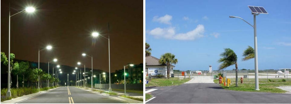
Examples of street lighting, including solar powered fixtures
