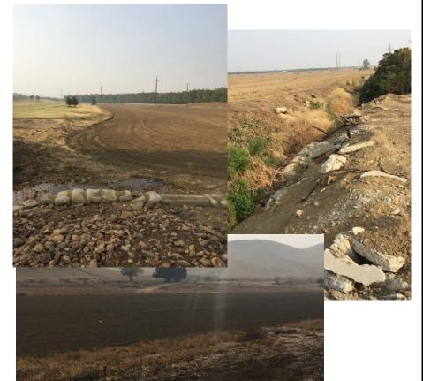
Photograph 26 - Drainage. Top-left and bottom: drainage graded/maintained by owner. Top-right, un-maintained, relic debris.
