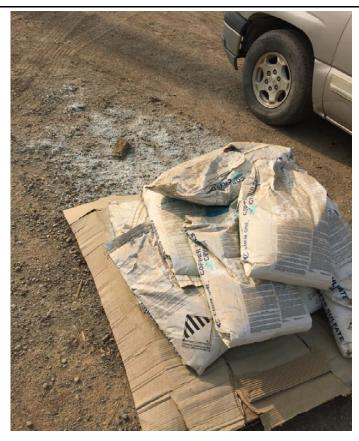
Photograph 12 - Improperly stored copper sulfate sacks potentially exposed to wind and rain runoff.
