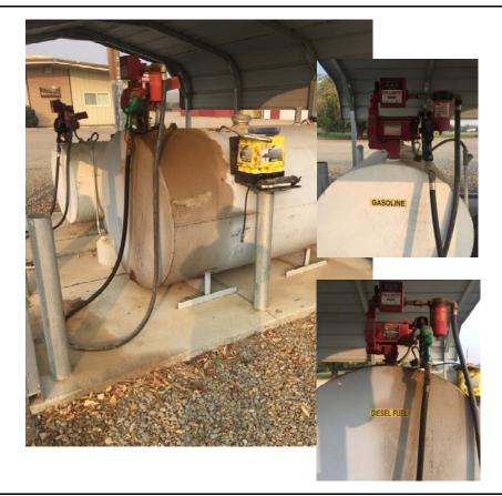
Photograph 2 - Fuel Storage Area, two ASTs, one diesel and one gasoline (outside subject property).
