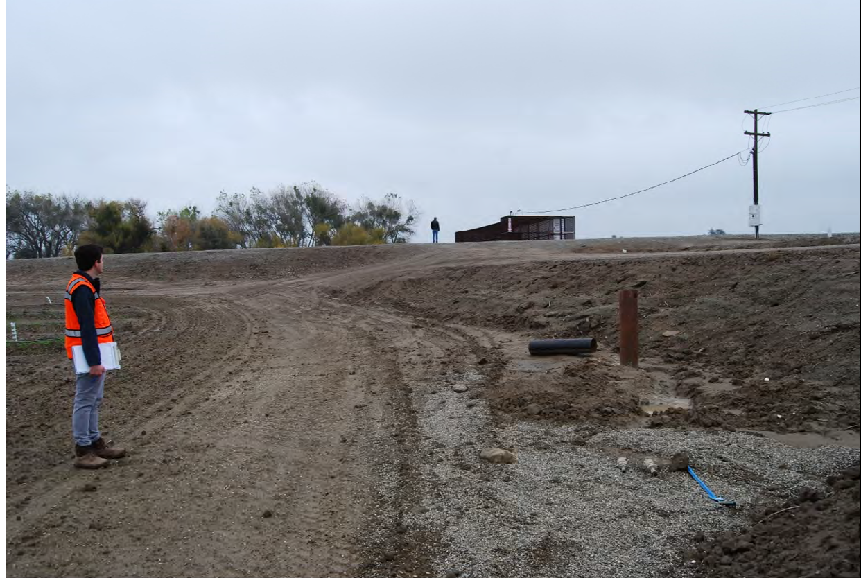
Borehole #2. View to the east toward San Joaquin River levee (ridge background) and Pescadero Ranch river water intake pumping station (caged facility in background).
