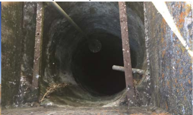
View down hand-dug well (parcel APN 001-011-031).
