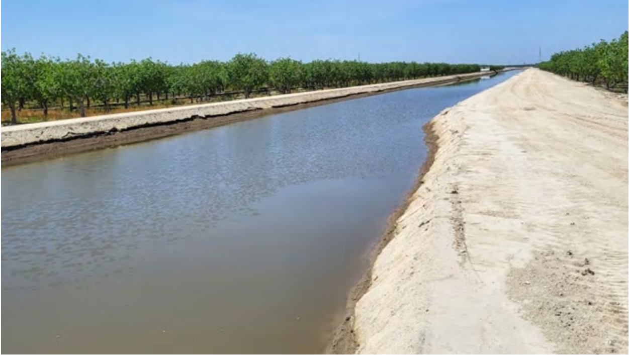
Water in an unlined canal conveyance system with pistachios orchards on either side.
