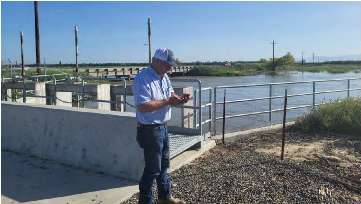
Mr. Cameron, using his computer telemetry to control the height of the turnout flood gates.
