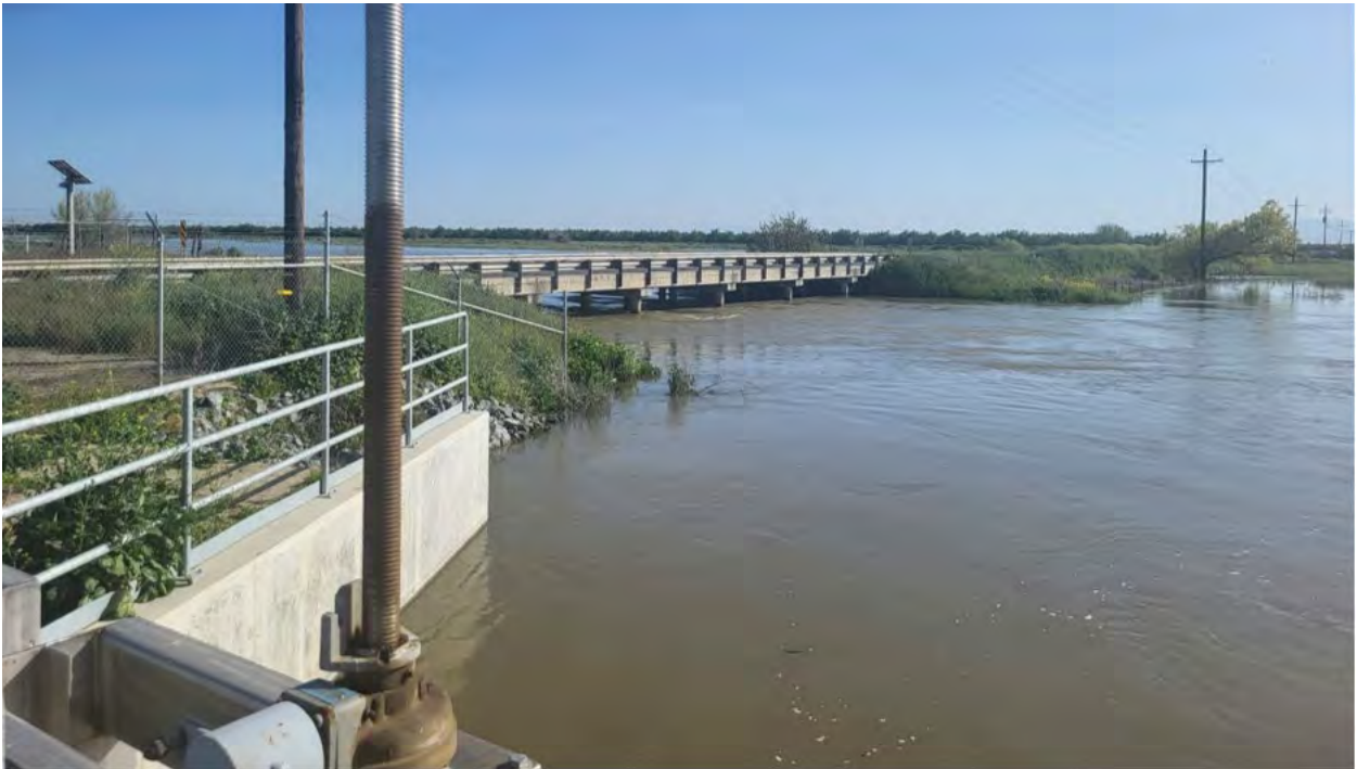
The diversion point of water on the Kings River North Fork canal into the Terranova Ranch.
