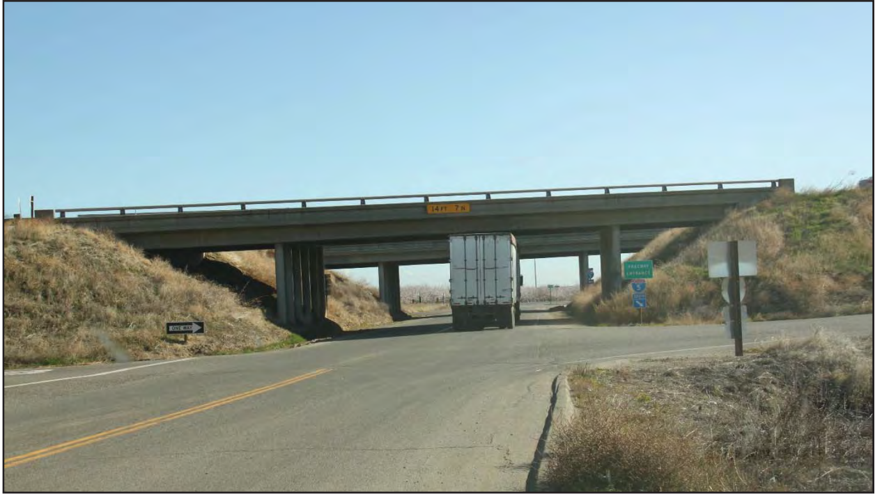
Fink Road / I-5 Interchange
