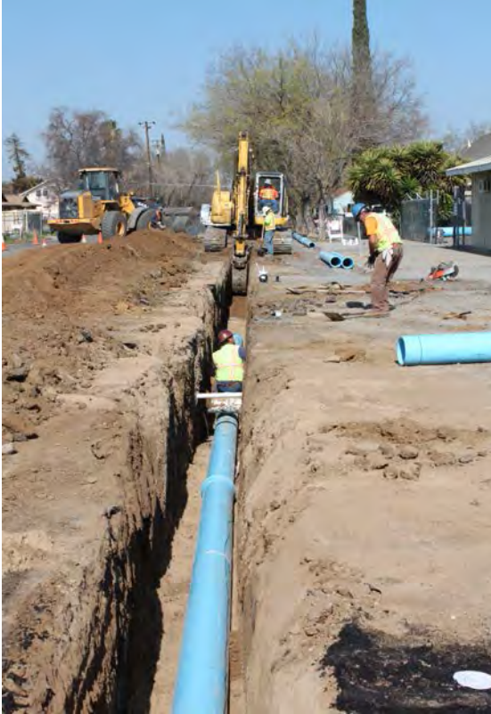
Photos reflect the water main replacement as part of the Fourth Street Infrastructure Project.
