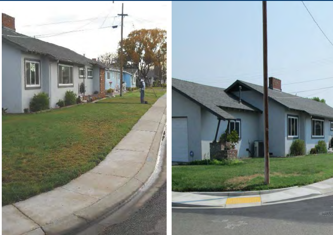
Photos reflect before and after ADA ramp improvements within the project area.
