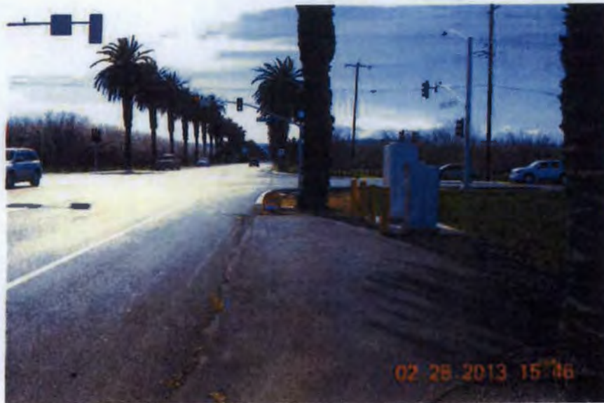
Northeast facing Southwest of the Intersection
