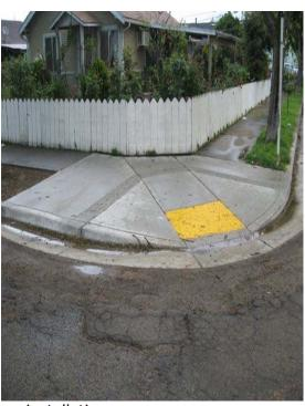
Photos reflect 3<sup>rd</sup> Street ADA accessible ramp installations.
