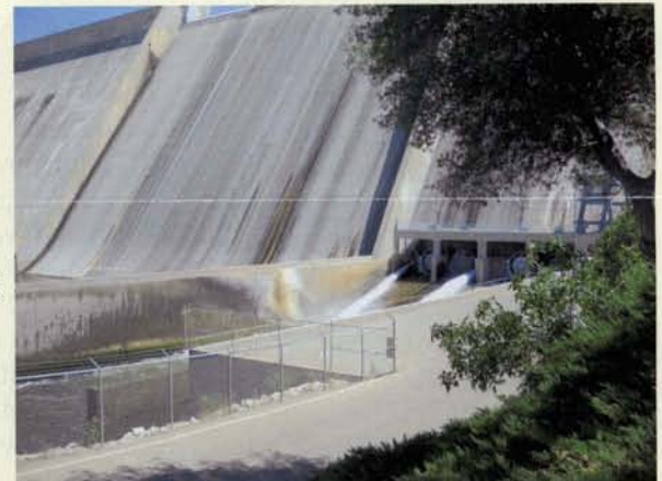
Water releases from Friant Dam switch from one large valve to two smaller valves as Interim Flows decrease from 800 cubic feet per second to 350 cfs on June 8, 2010
