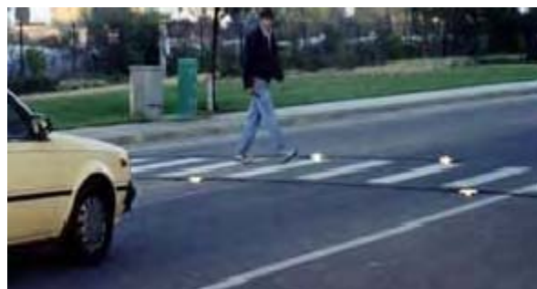
Figure B-25: In-Roadway Warning Lights
