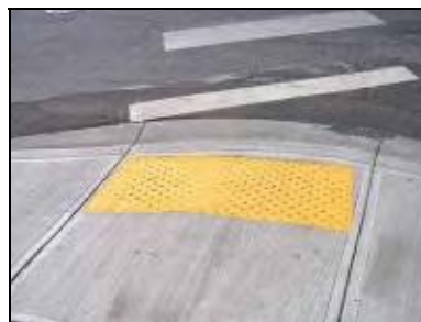
Curb ramp with truncated domes
