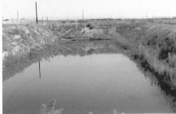
Pilot Recharge Basin
